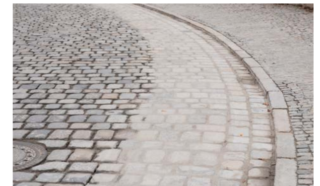
Barrier-free pavement repair with MORTAR MIX in Amberg, Germany
