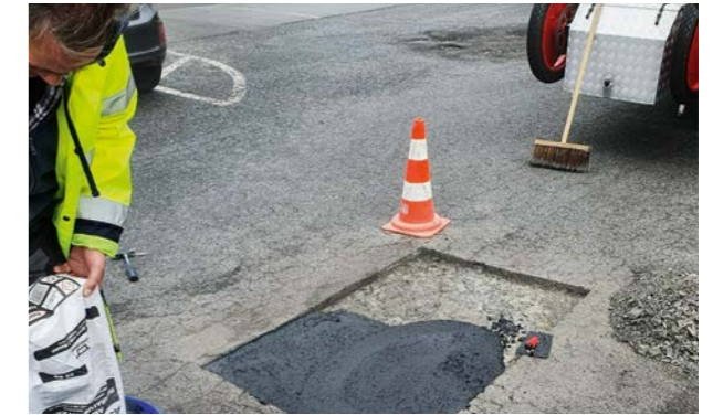
Repair of parking lot with ASPHALT REPAIR MIX
