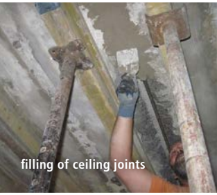
liquid-tight repair at gas station
