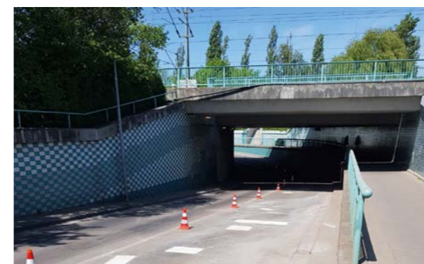
Repair of a concrete roadway with CONCRETE MIX in Frankfurt, Germany
