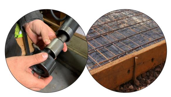
Unlike hammering the form stakes in, using the Drive Shim prevents mushrooming and splintering which can occur over time. The long-term cost saving of keeping these form stakes usable on multiple jobs is very positive for the industry.
